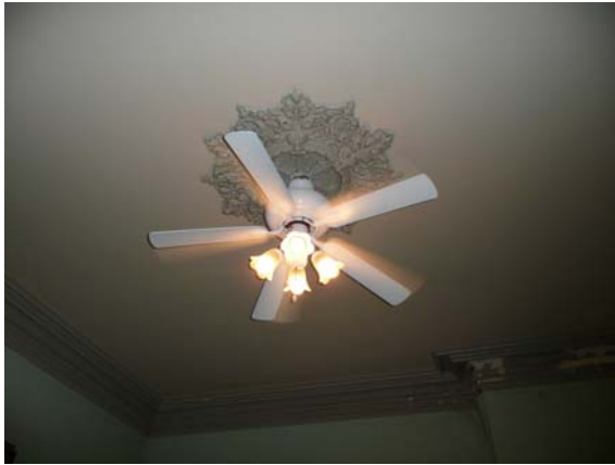
Detail of Lighting and Ceiling
