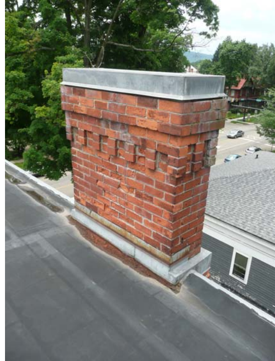
Chimney #1 – East and North Face
