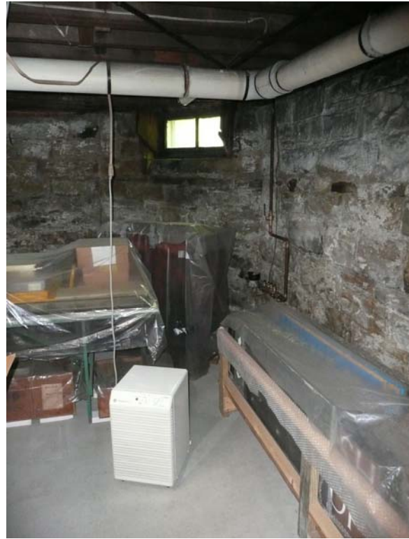
View of East and South Wall of Room
