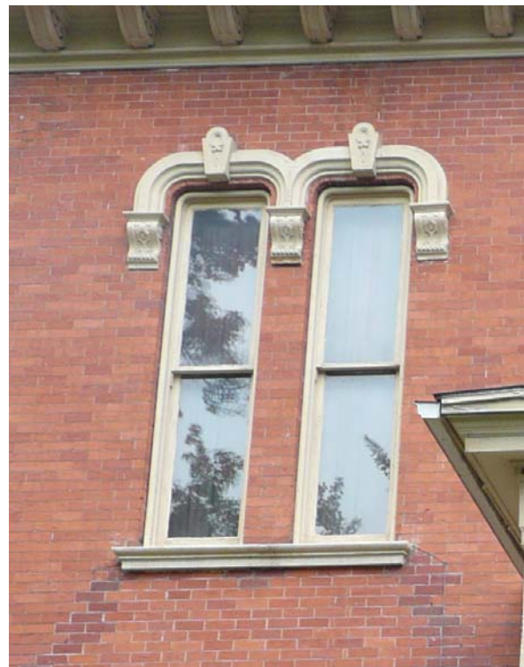
South Elevation – Second Floor (total of 3 pair)
