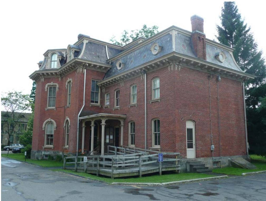
Overall View Looking Southwest
