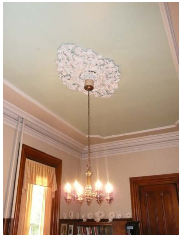
Detail of Pendant Light Fixture and Ceiling
