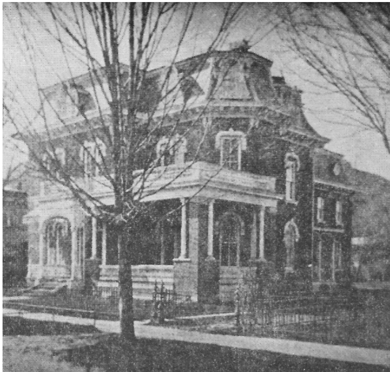
Undated photo showing Colonial Revival porch
