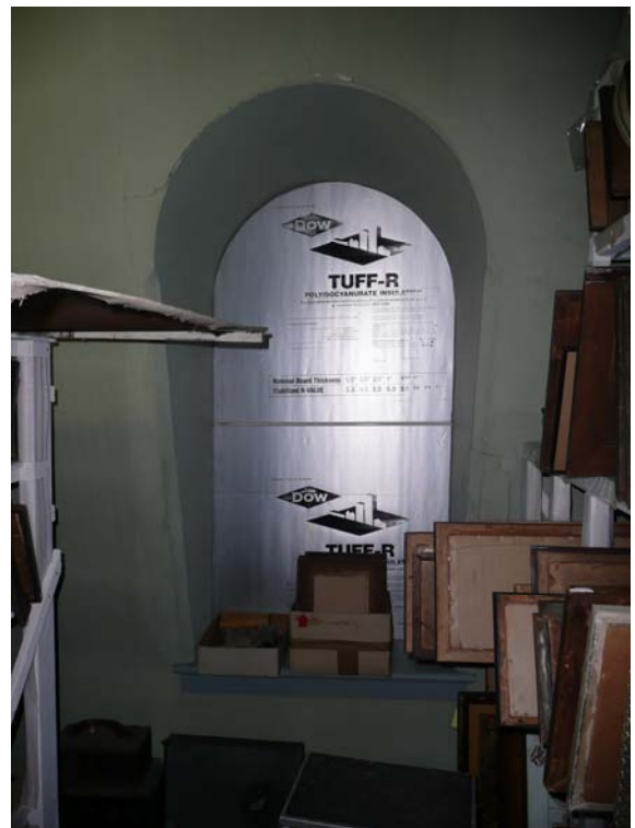
Detail of Dormer Window facing West
