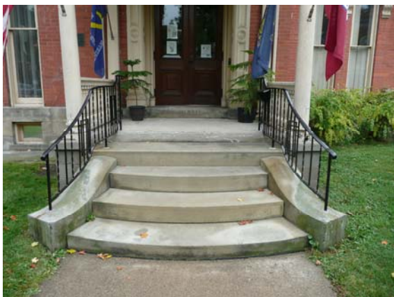
Close-up View of Stone Steps
