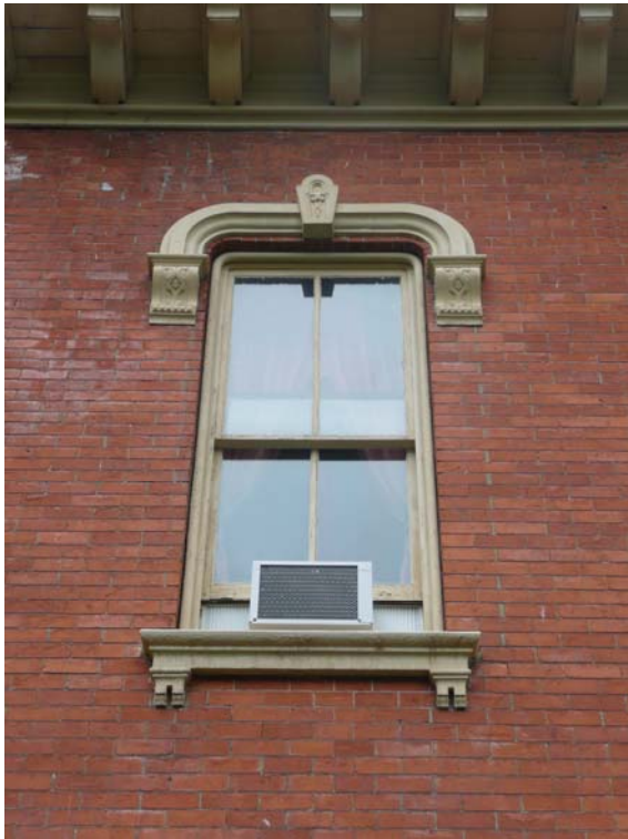
Window AC Unit at Photo Collections 203
