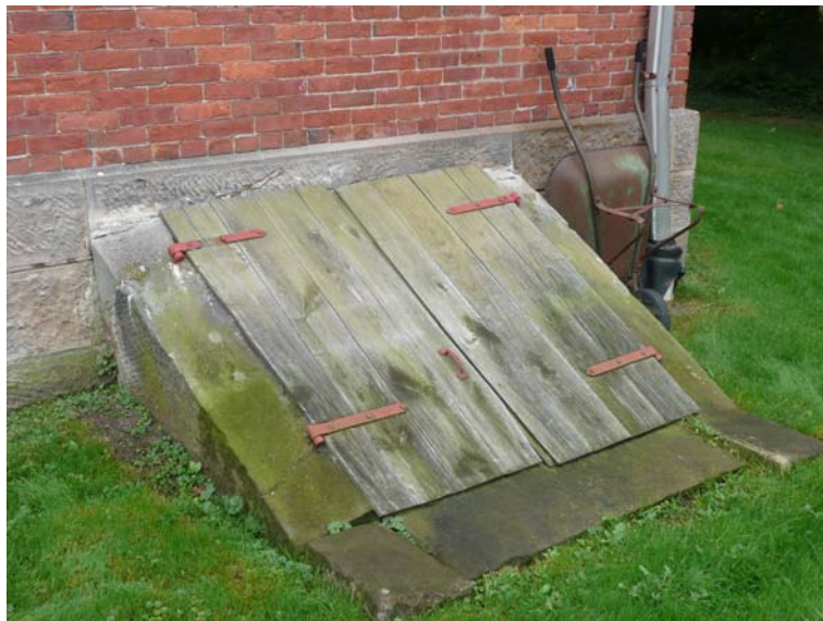
Exterior Entrance to Basement
