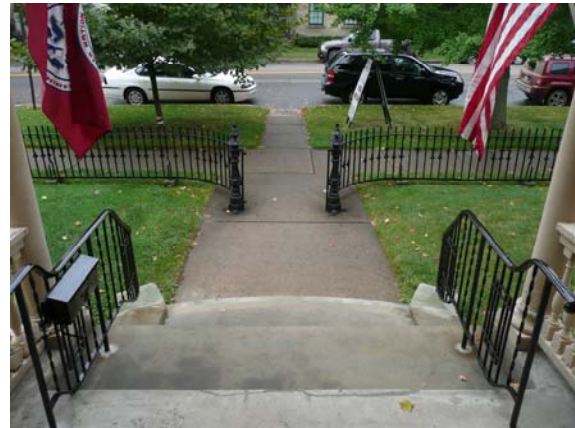
Concrete Walkway from Building Entrance to Street
