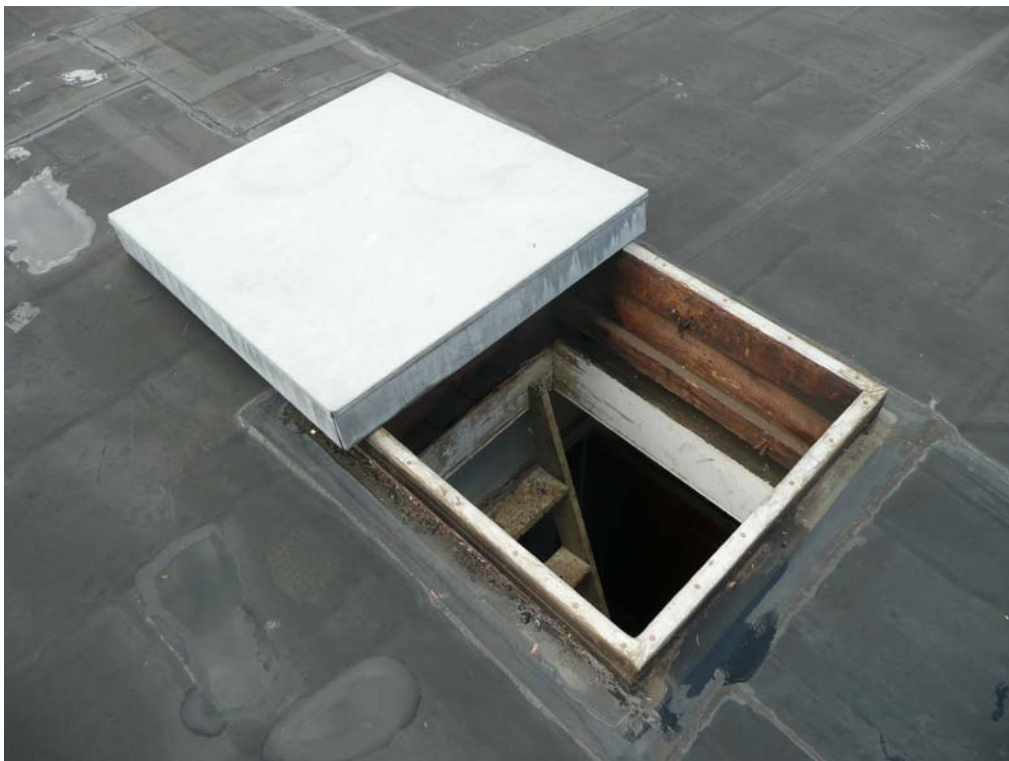
Roof Access Hatch at Front Roof
