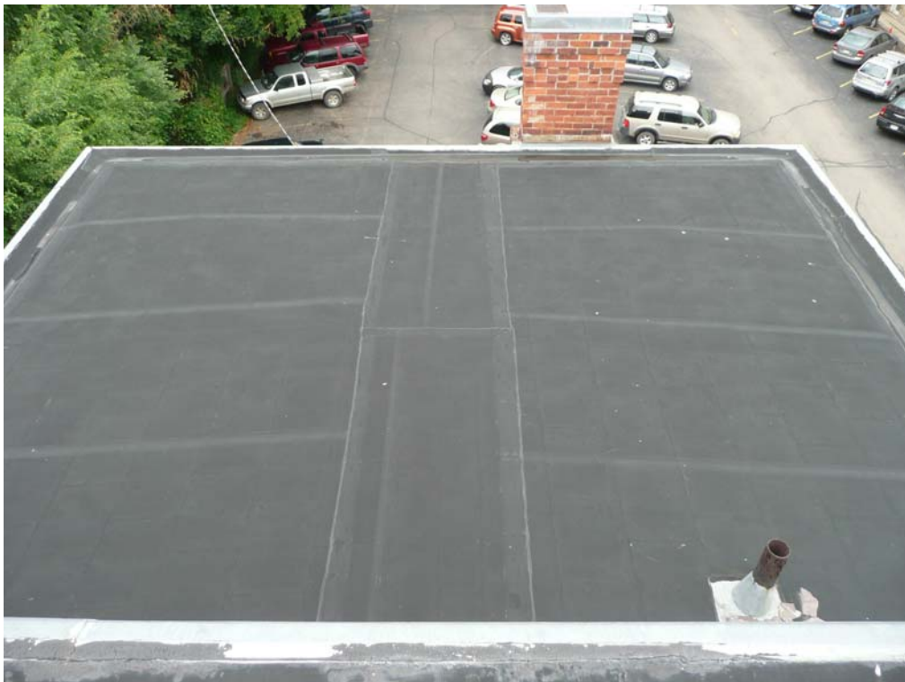
View Looking North at Rear Roof from Front Roof
