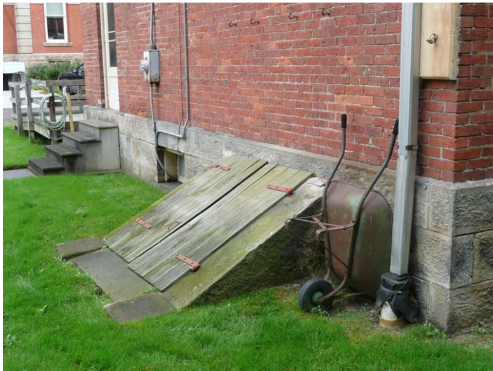
Typical Stone Foundation and Brick at Rear of House
