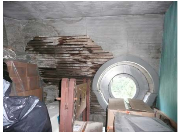
View Looking West
