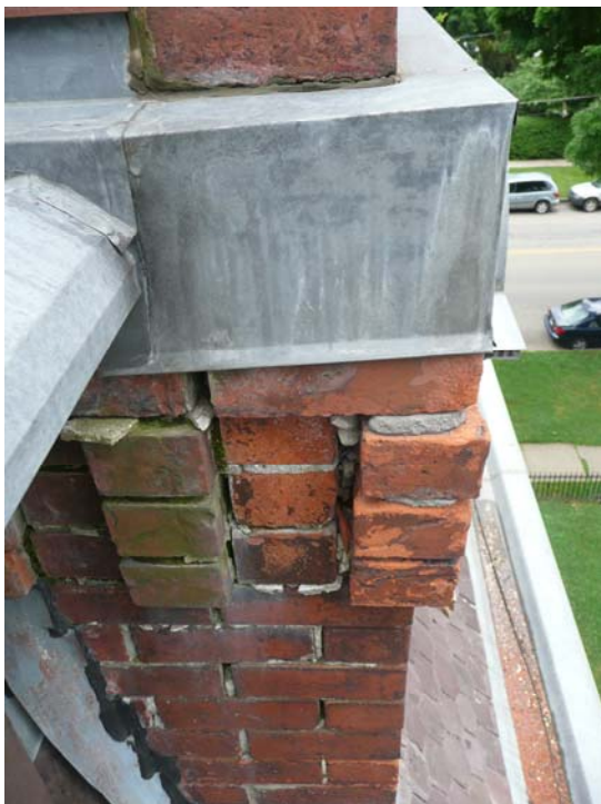
Chimney #1 – Detail of North Face
