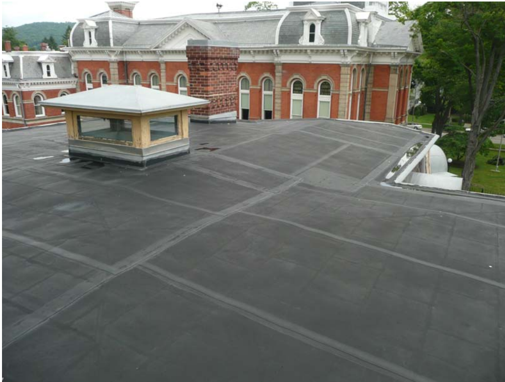
View Looking East from Southwest Corner of Front Roof
