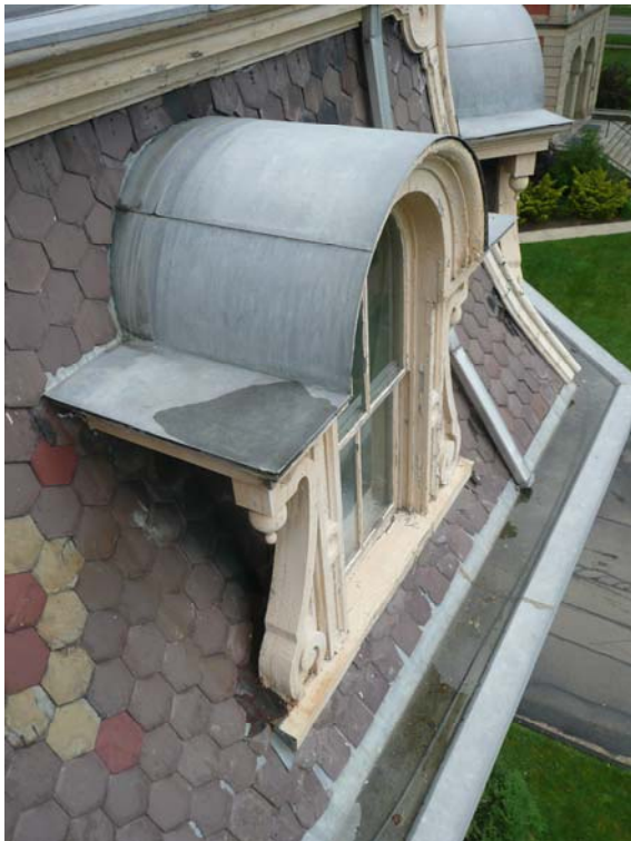
Overhead View of Typical Front Roof Dormer (south)
