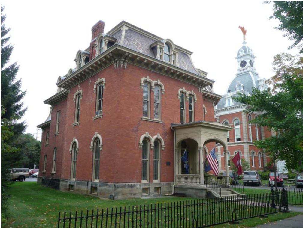
Overall View of Looking Northeast
