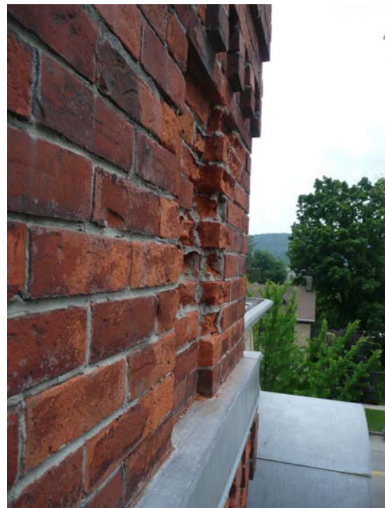
Chimney #1 – Detail of West Face
