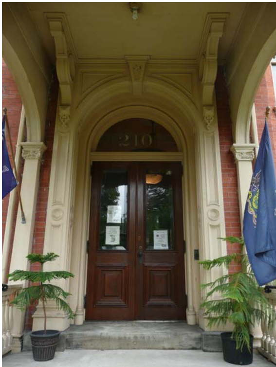
Front Doors with Arched Transom Window
