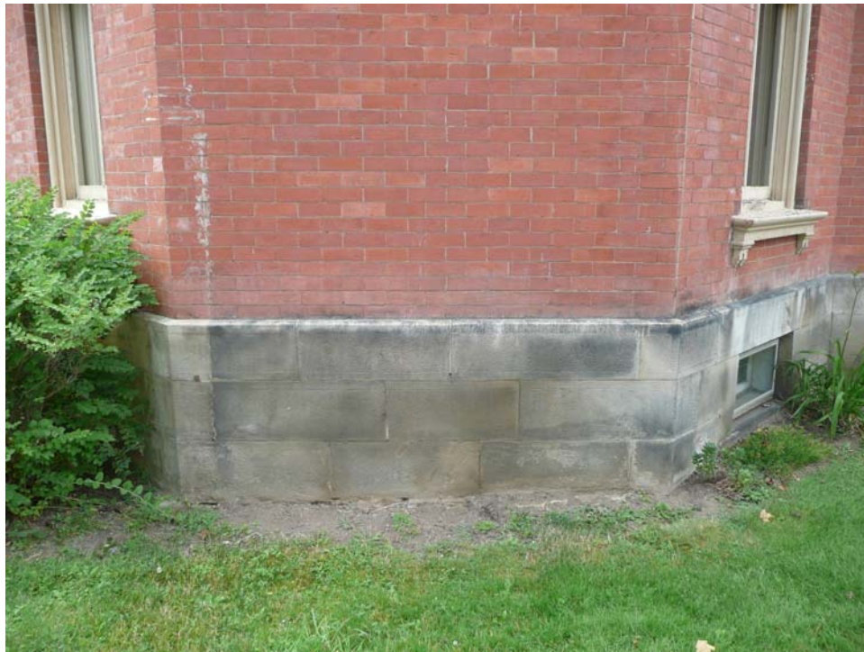
Typical Stone Foundation and Brick at Front of House
