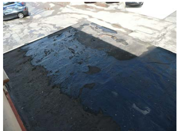
View of Porch Roof from Second Floor Window
