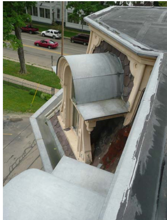
Overhead View of Typical Front Roof Dormer (east)
