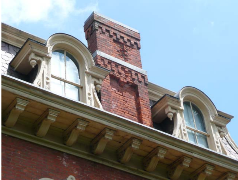
Typical Dormer at Front Roof (total of 8)
