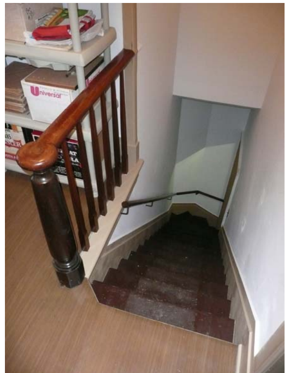
View Down Stair to First Floor
