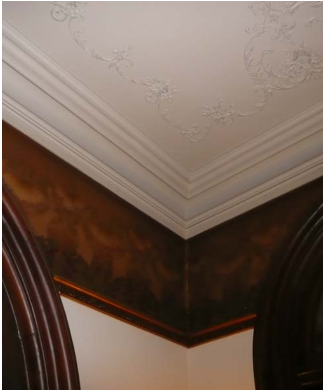
Wall and Ceiling Detail
