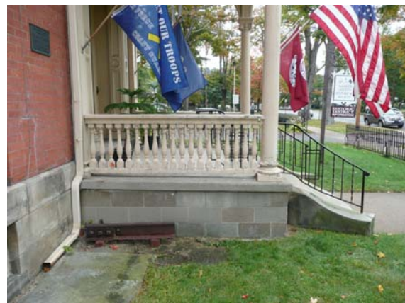
Close-up View of CMU Foundation
