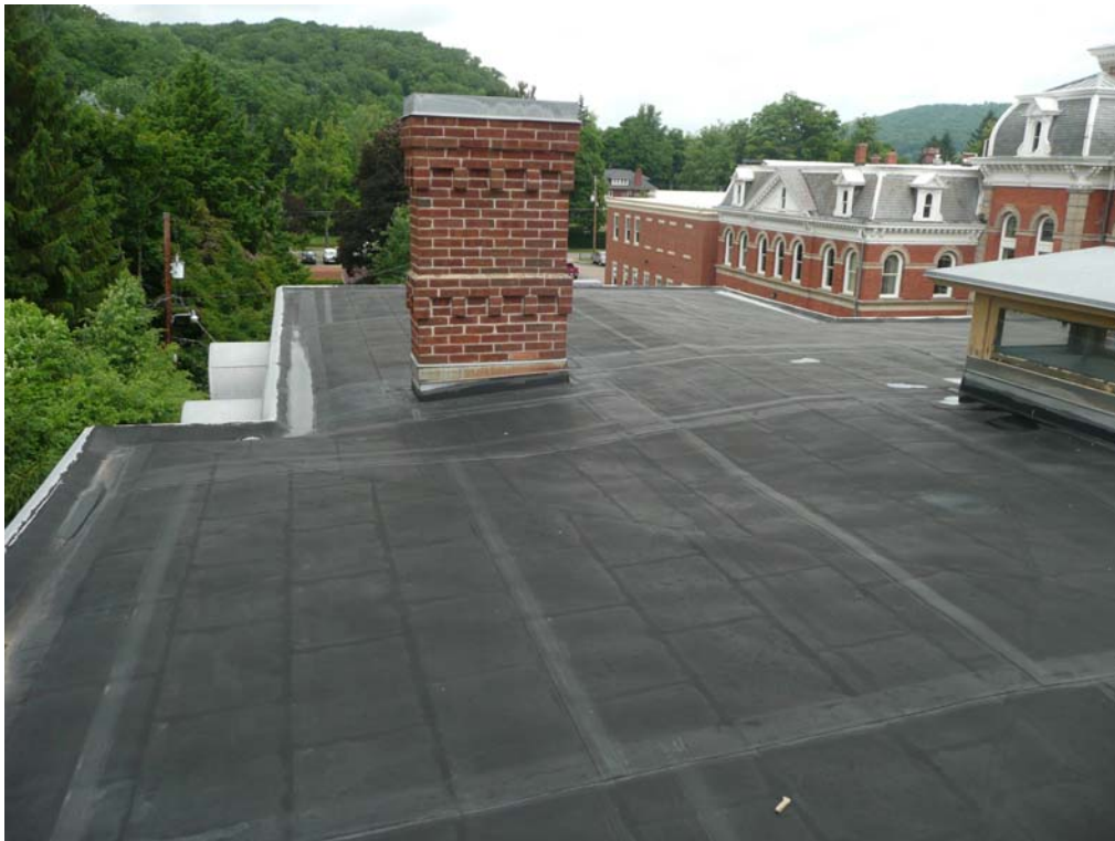
View Looking North from Southwest Corner of Front Roof
