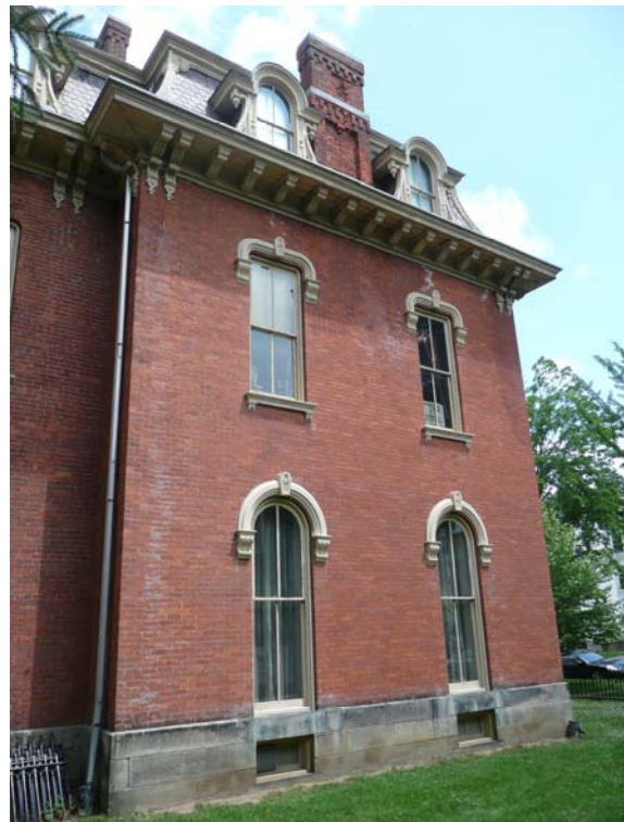
Partial West Elevation
