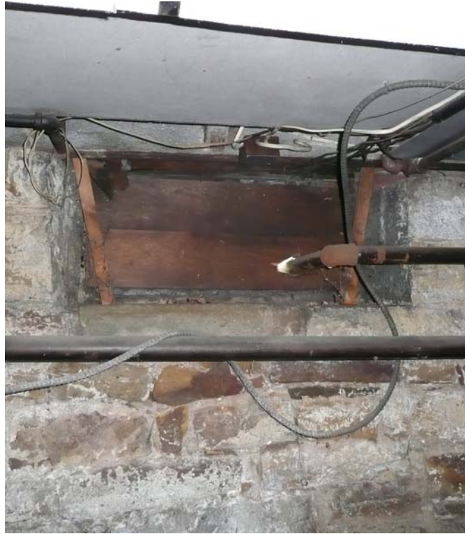
Detail of Infilled Window facing East
