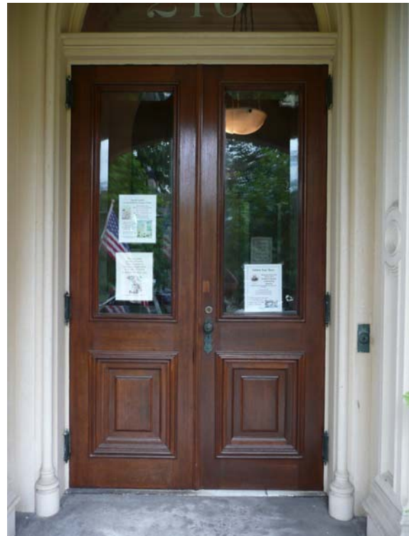
Detail of Front Doors
