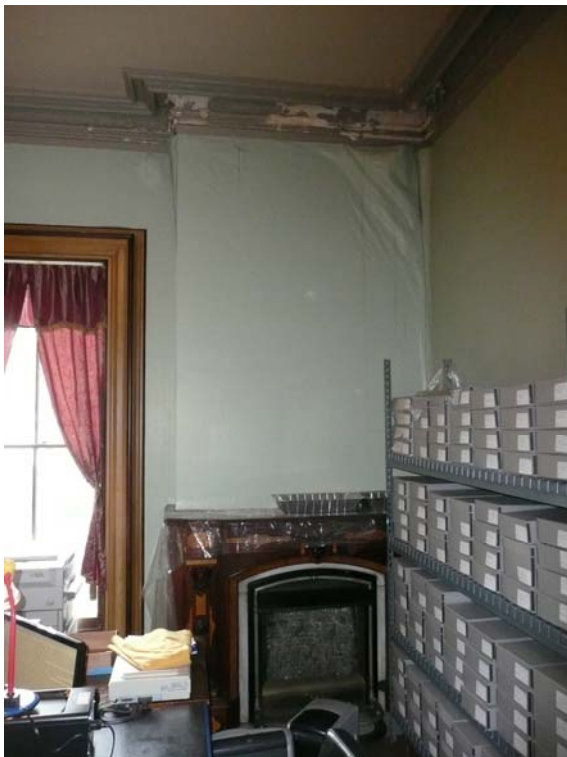
View Looking West at Fireplace
