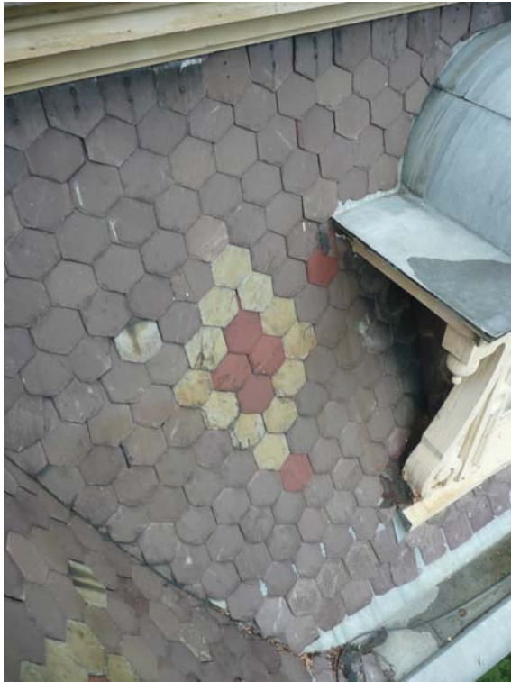
Multi-color Slate Detail at Front Roof
