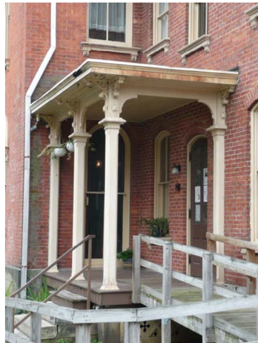
View of Porch 2 Looking South
