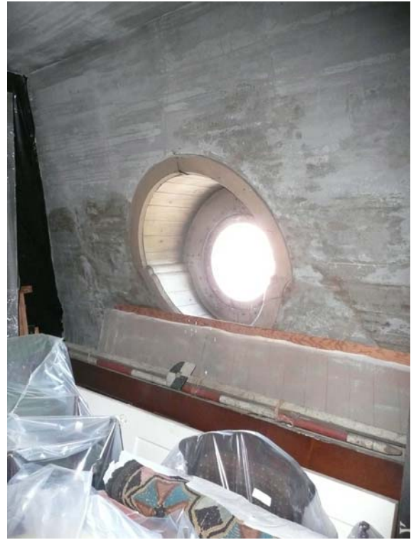
View of East Wall
