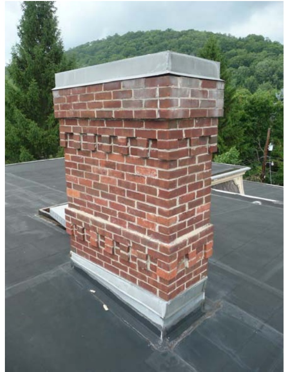
Looking Northwest at Chimney #3
