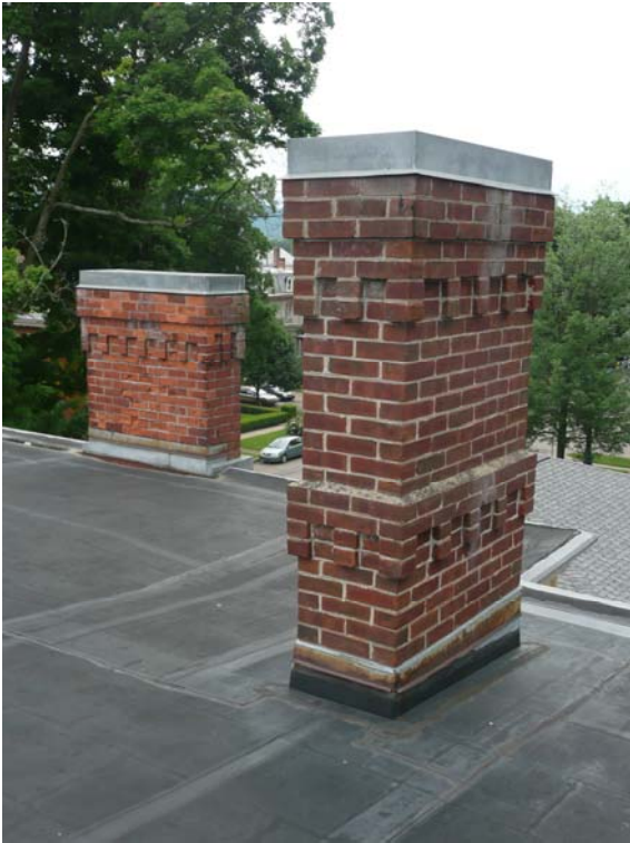
Looking West at Chimney #2 (Chimney #1 in background)
