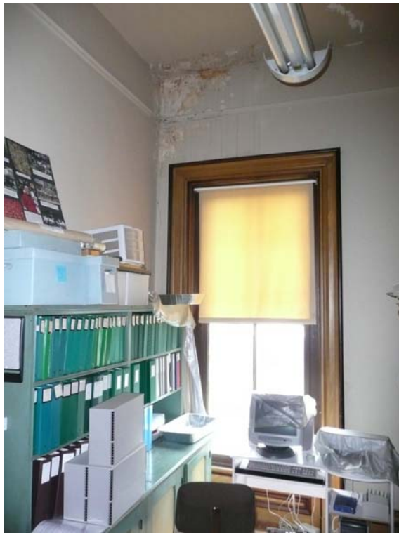
View Looking West
