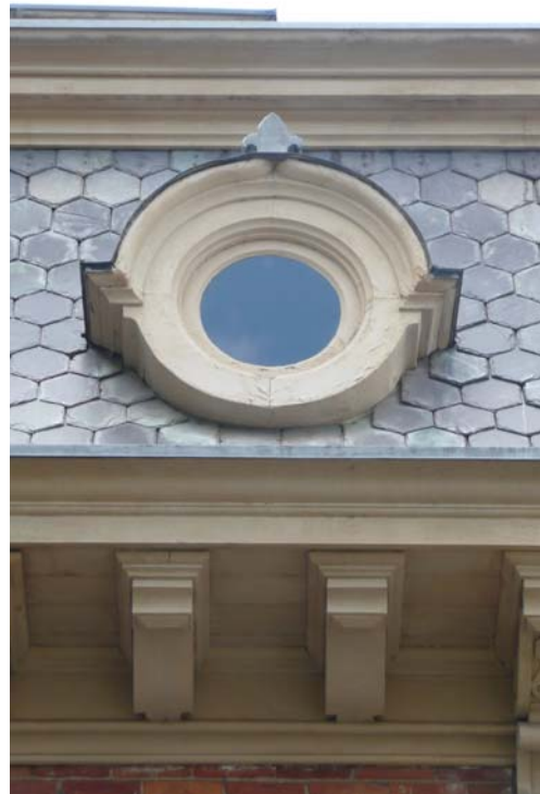
Typical Dormer at Rear Roof (total of 5)
