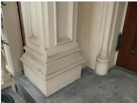
Detail of Recessed Door Frame
