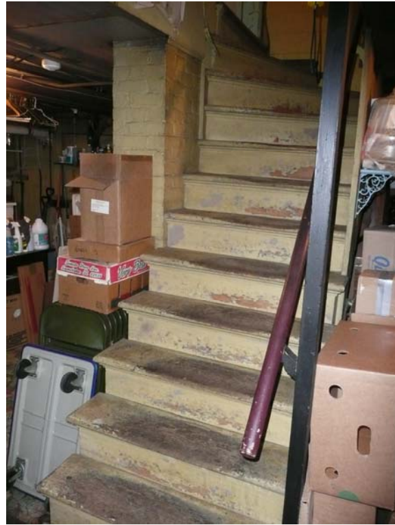
View of Stair to First Floor
