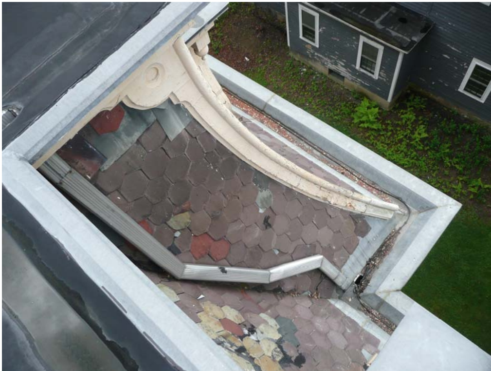
View of Northeast Corner of Front Roof
