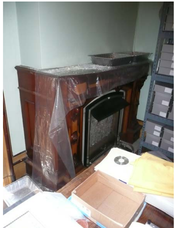
Detail View of Fireplace
