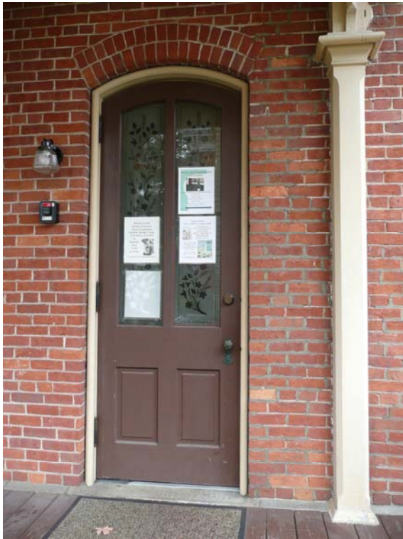
East Entrance at Porch #2
