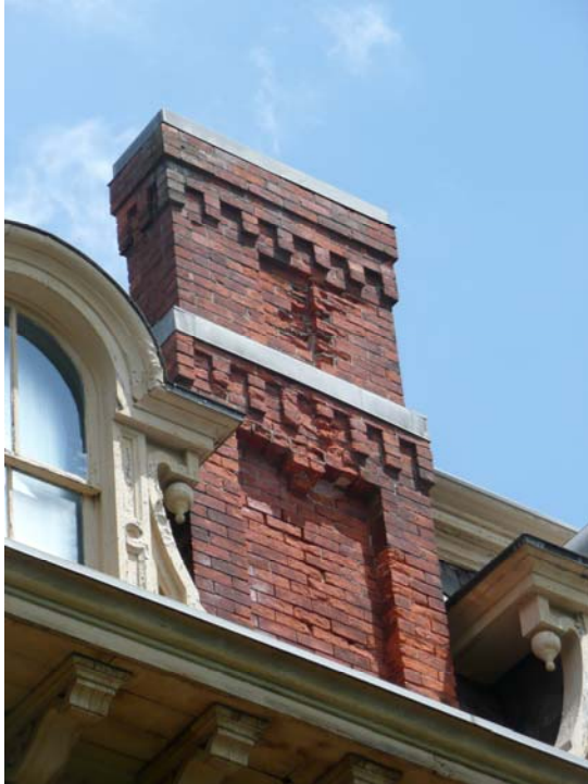
Chimney #1 – West Face
