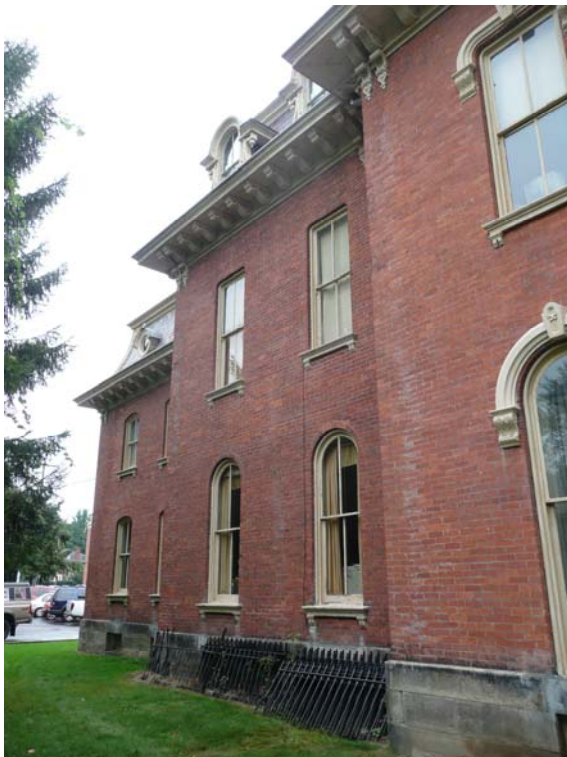
Partial West Elevation
