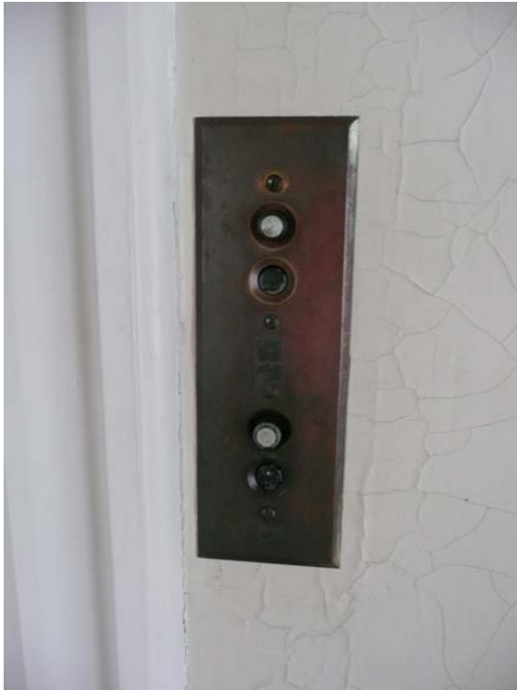
Light Switch at Parlor 104
