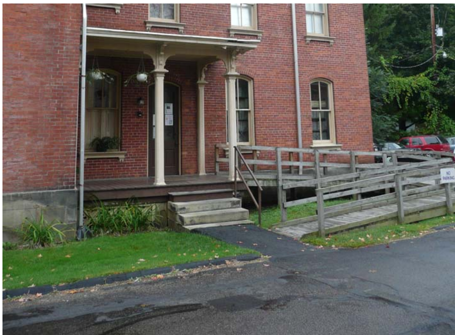
Asphalt Walkway to Side Entrance
