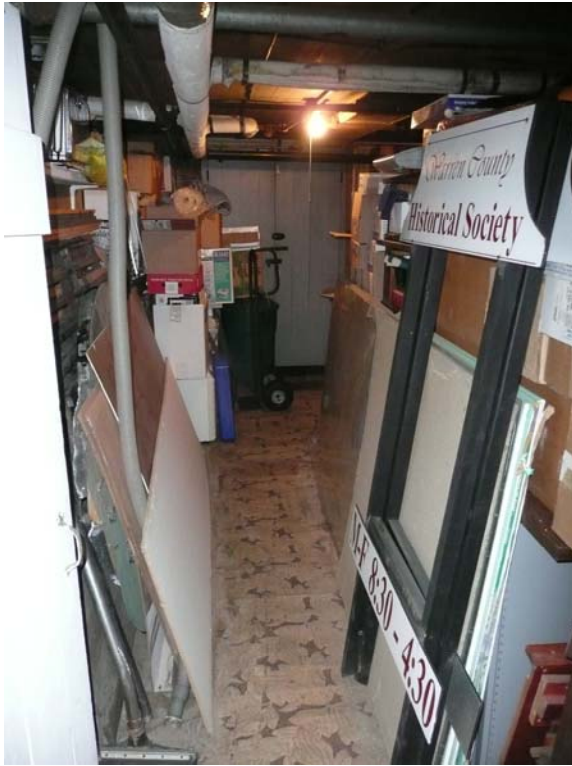
View Looking North at Doors to Exterior Stair
