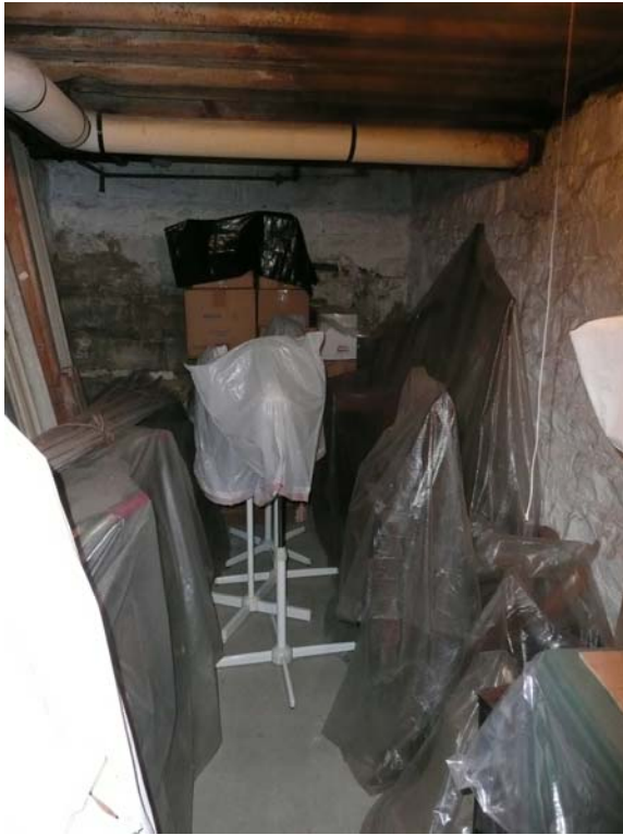
View Looking South
