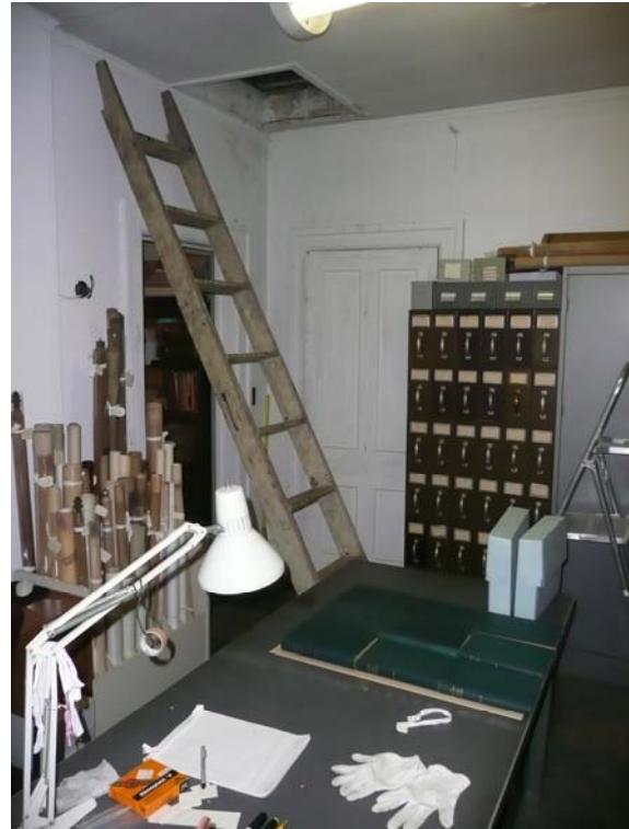
View Looking West at Roof Access Hatch
