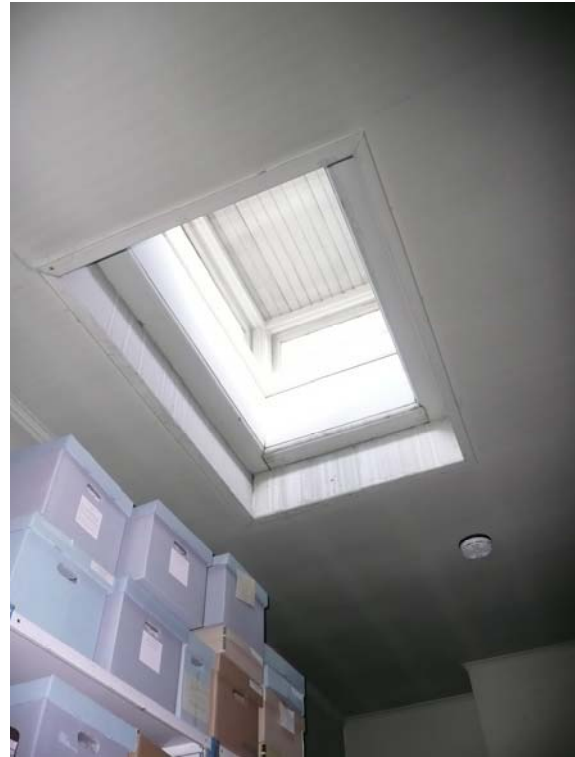
Detail of Skylight
