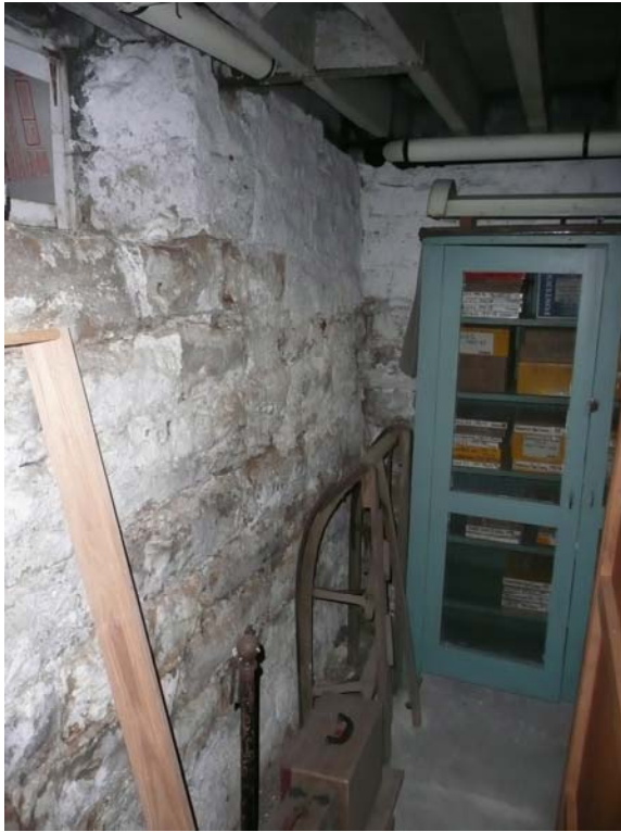
View of Southwest Corner of Room
