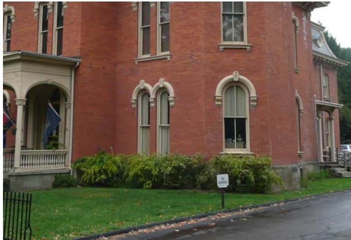
View of Landscaping
