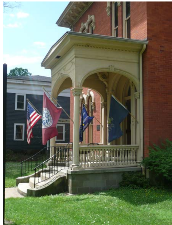
Front Entrance Porch looking West
