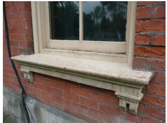
Typical Cast Iron Sill
