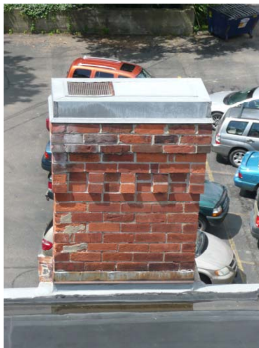
Looking North at Chimney #4
