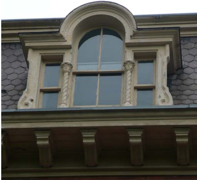
Unique Dormer at West Elevation on Front Roof (only one)
