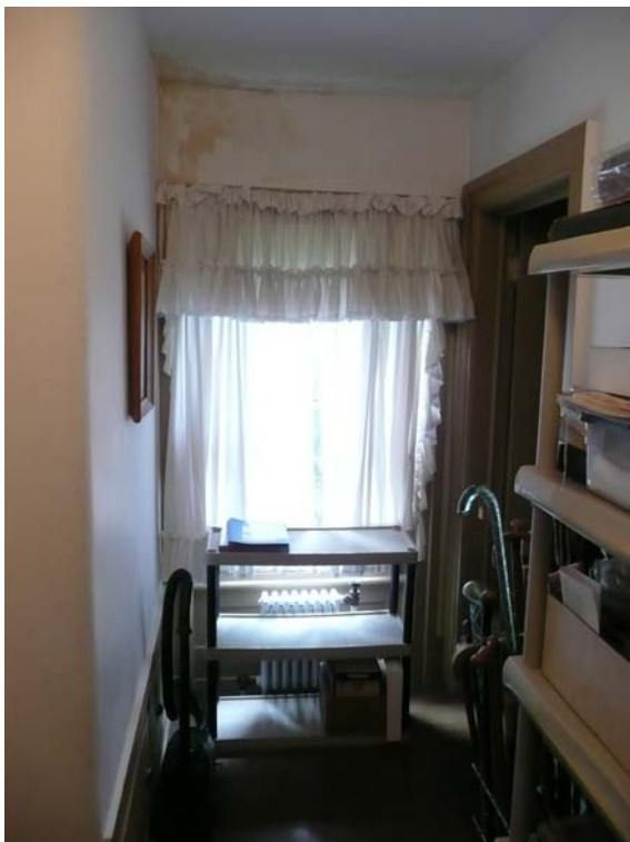
View Looking West
