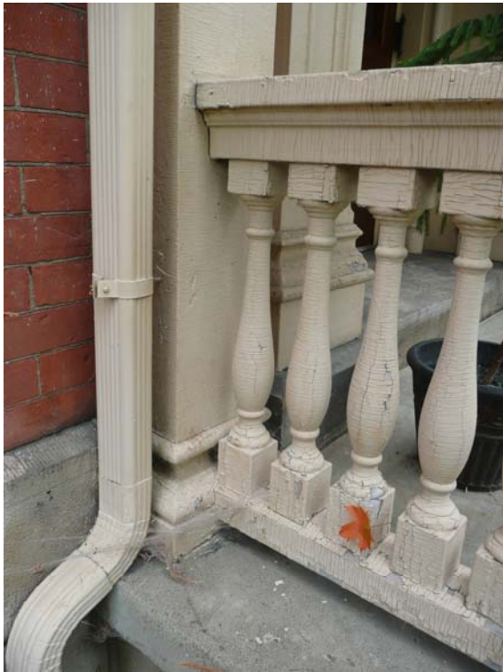
Detail of Railing and Pilaster
