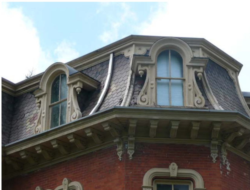
Typical Dormer at Front Roof (total of 8)
