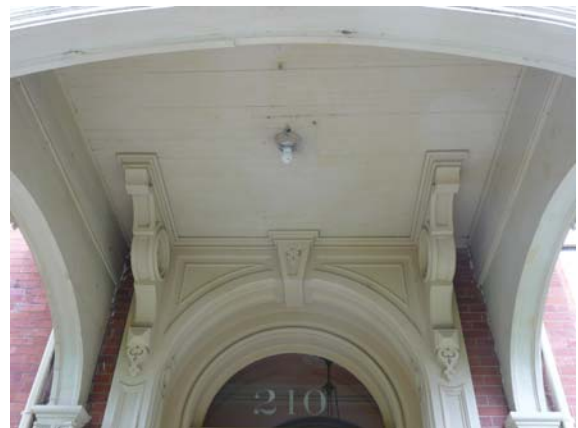
Detail of Door Frame and Brackets
