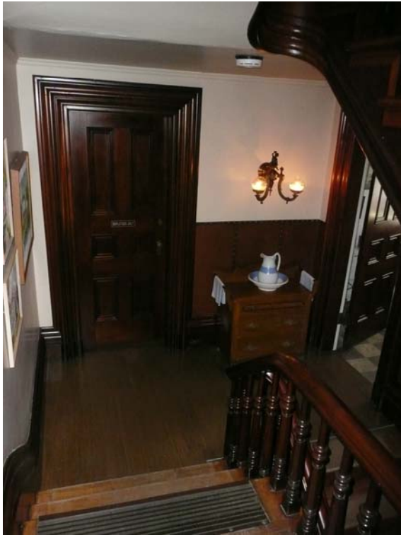
View Looking North at Stair Landing
