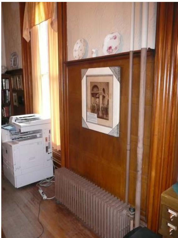
View of West Wall
