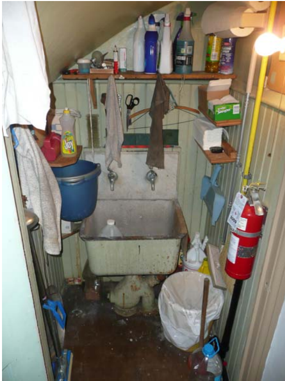
View of Utility Closet
