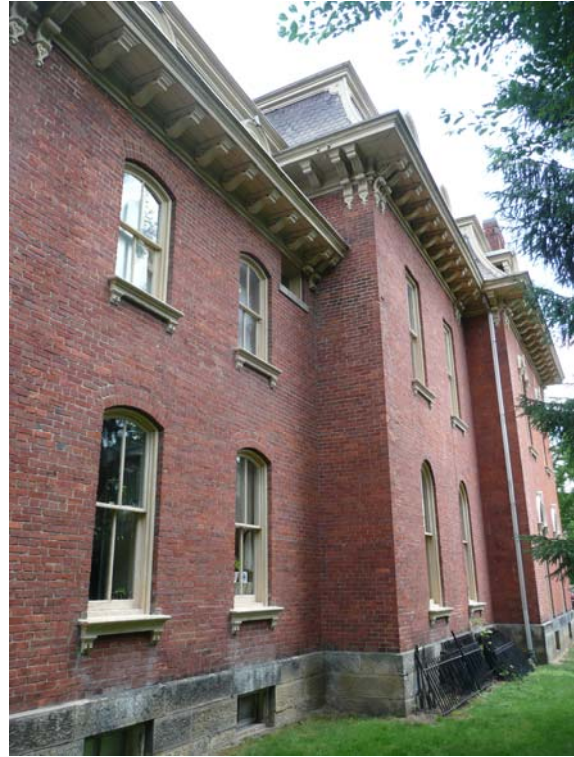
Partial West Elevation
