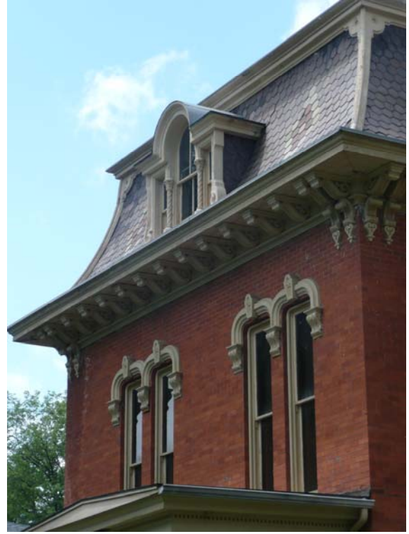
Detail of South Elevation
