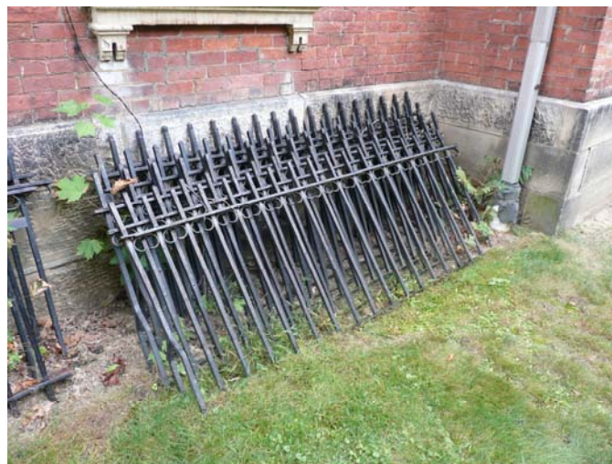
Extra Fence Sections along West Wall of House
