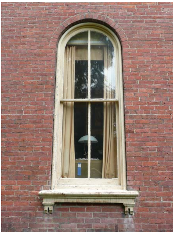
West Elevation – First Floor Middle (total of 2)
