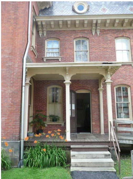
View of Porch 2 Looking West
